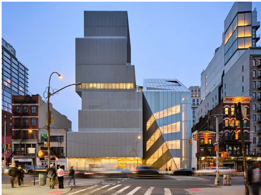
The facade of the new New Museum. Photography by Jason Keen.
